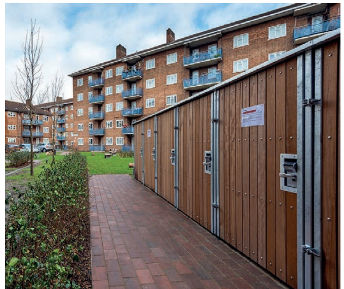
Figure 82 Bike storage buildings provided adjacent to apartment around Brunstane Square
