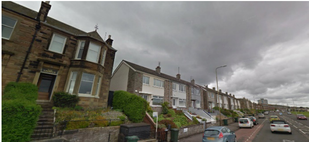
Figure 23 – New terraced houses to East of site on Seaview Terrace
