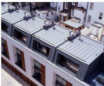
Figure 20 – Zinc Mansard Roof
