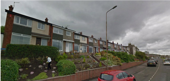
Figure 24 – New terraced houses to East of site on Seaview Terrace
