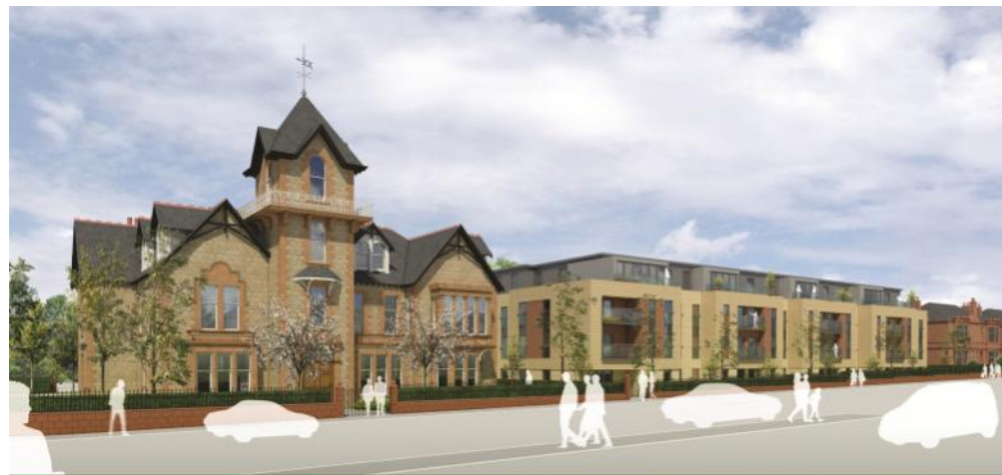
Queensferry Road, Barnton - Complete
