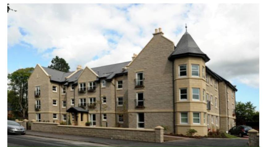
Caiystane Court, Firrhill - Complete
