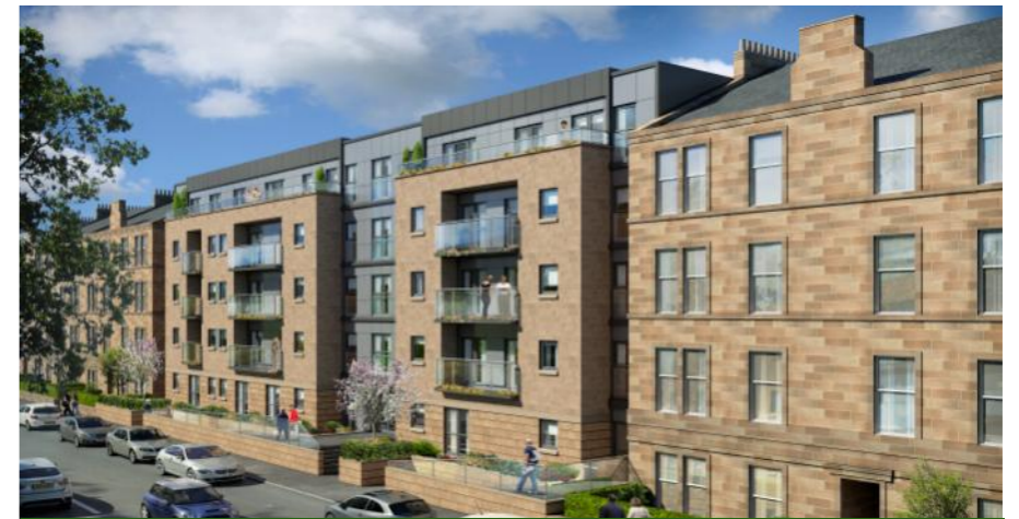
Balcarres Street, Morningside - Under Construction
