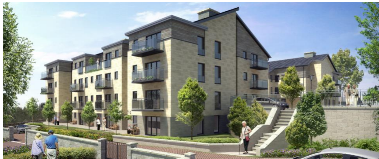
Isla Road, Perth - Under Construction
