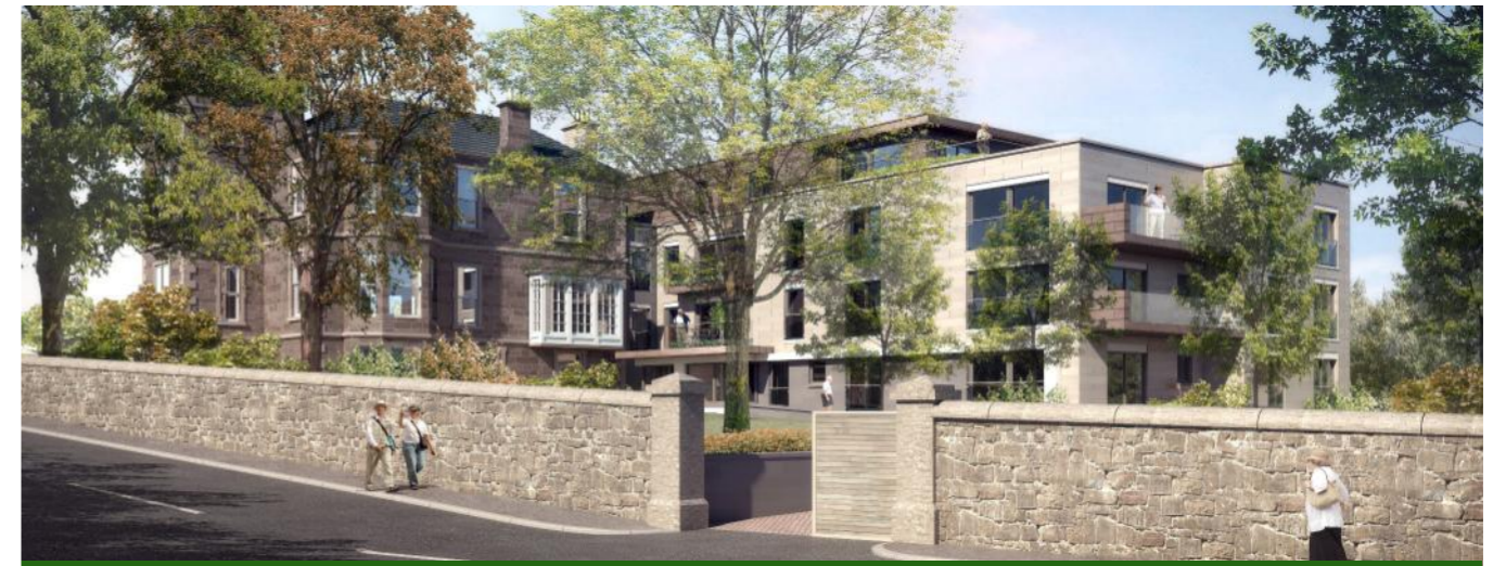
Murrayfield Road, Edinburgh - Under Construction
