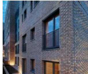
Iron Railing Ballustrades
