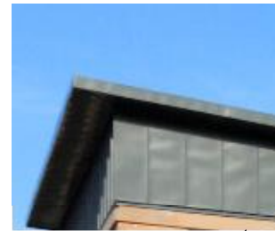
Zinc Butterfly Roof
