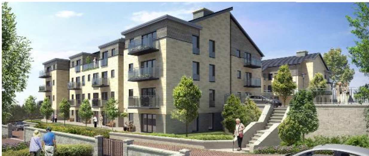
Isla Road, Perth - Under Construction
