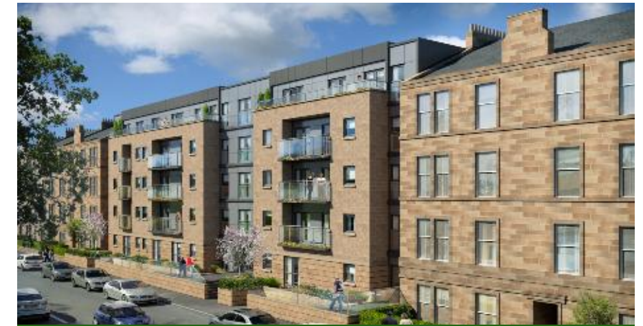
Balcarres Street, Morningside - Under Construction
