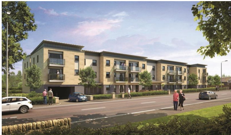
Liberton Road, Edinburgh - Under Construction
