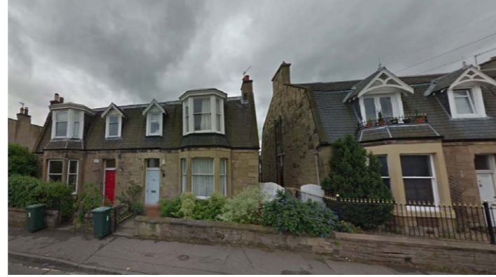
2 to 8 Milton Road East
