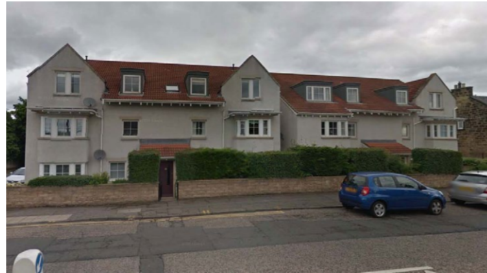
11a & 11b Milton Road East
